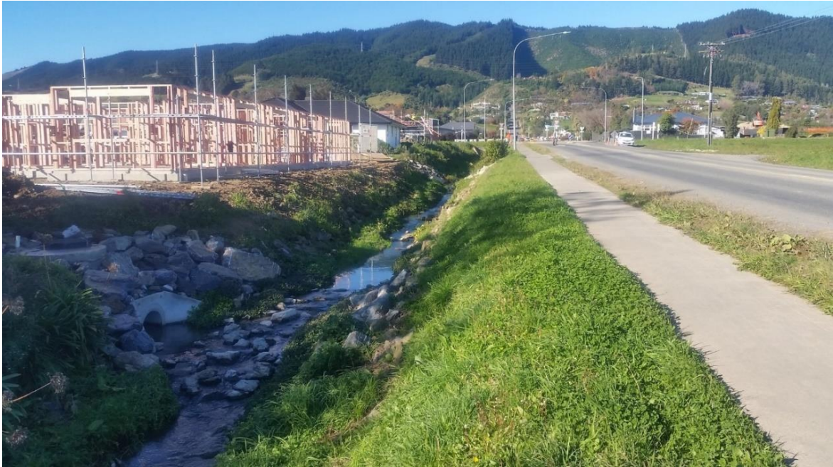
Figure 2: Lack of adequate river setbacks (Bateup Road)-
