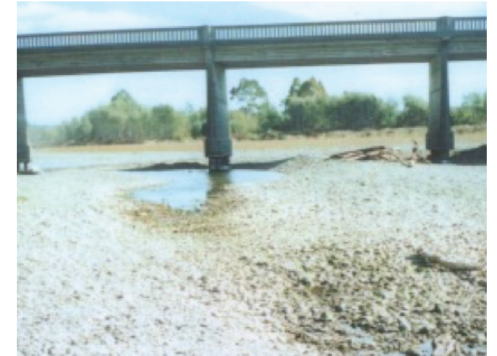
Waimea River at the Appleby Bridge in drought in February 2001
