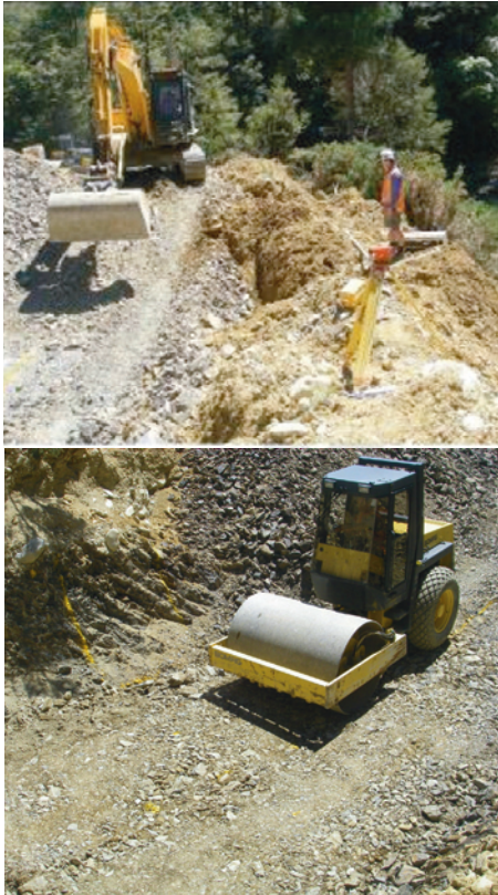
Figure 3: Excavation of trenches on site and compaction trials
