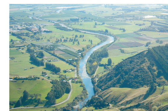
Looking out over the Wairoa Gorge – Waimea East Irrigation Intake in the foreground on the right
