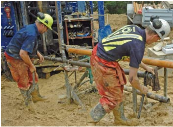
Drillers remove core samples.
