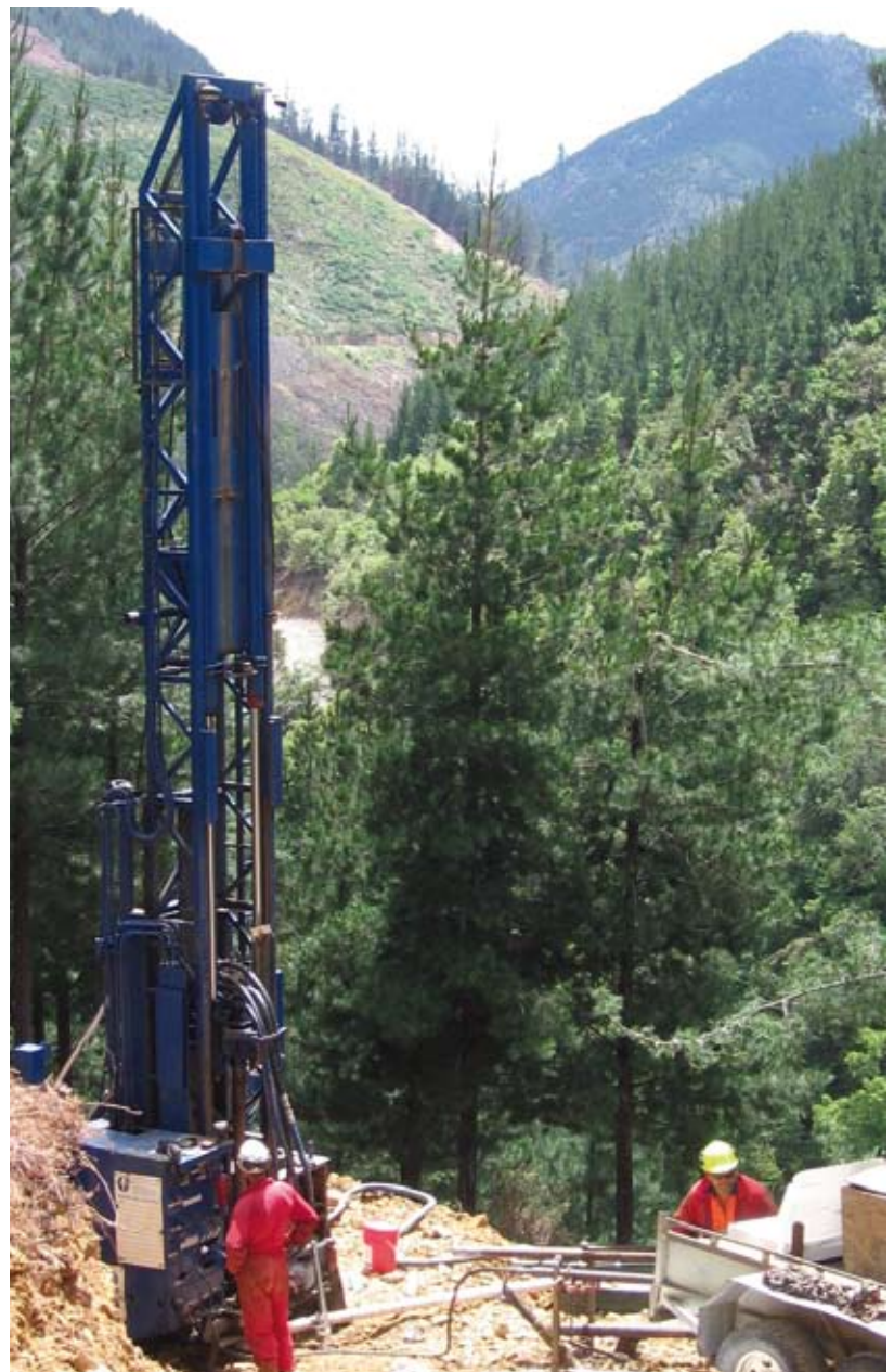
Drillers on site in the Lee Valley.
