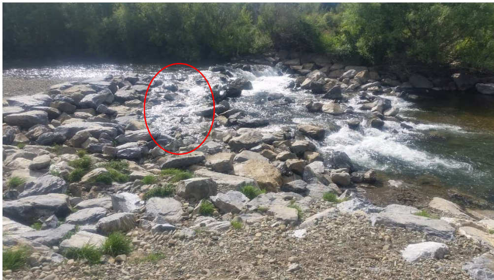
Wai-iti Weir 2 about 100m downstream of Waimea West Rd in November 2017. Note the concreted ramp (circled) provides a channel with lower water velocities and less turbulent flow. This ramp now needs to be extended across to the true right (towards the foreground of the photo).
