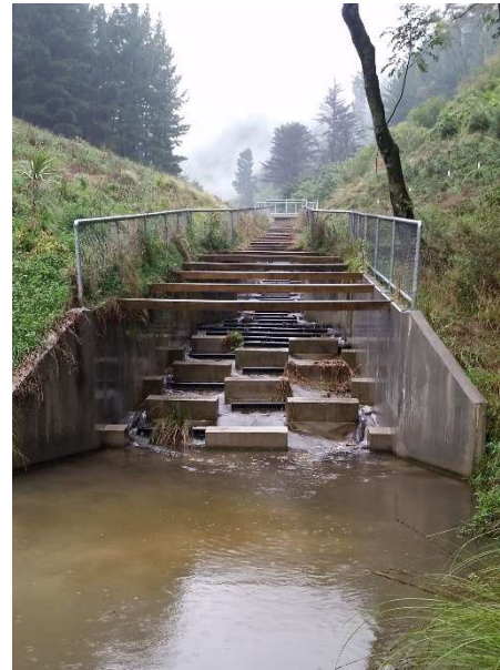
The spillway/fish pass on Reservoir Creek 2016
