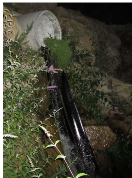
Left: Totaranui Rd Culvert 18 before a rubber apron and mussel spat rope were attached to encourage fish passage (Dec 2012). Right: With rubber apron attached to the culvert outlet (Jan 2014).
