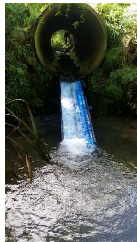
Left: Tower Road culvert with a rubber apron (February 2014). Right: With a floating ramp and baffles within the culvert (November 2016).
