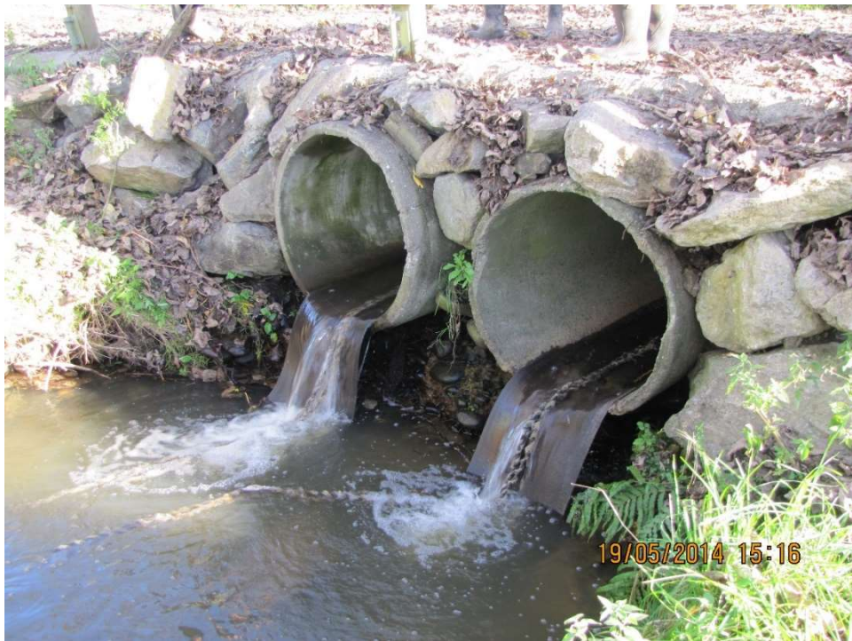
Teapot Valley Stream 1.1 km upstream confluence of Wai-iti River following fish passage remediation May 2014
