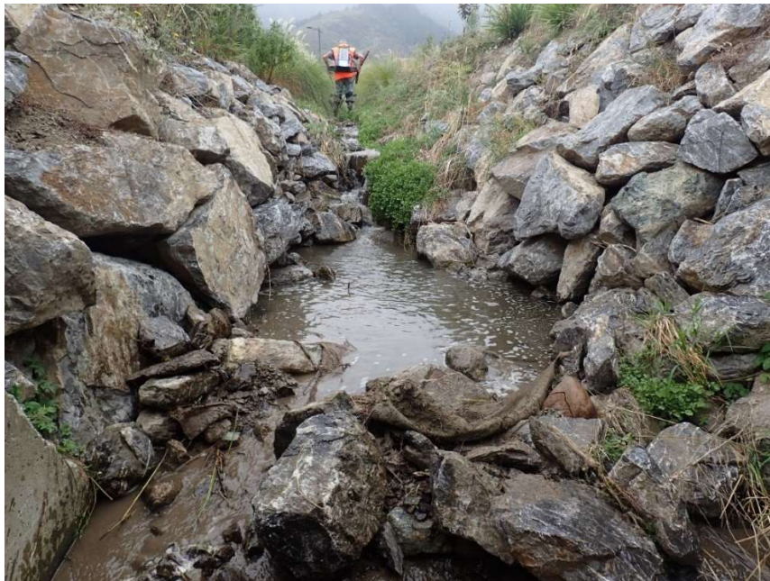
Reservoir Creek about 10m upstream of Hill St, March 2016.
