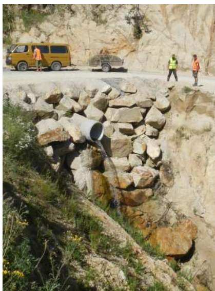
Left: Totaranui Rd Culvert 18 before a rubber apron and mussel spat rope were attached to encourage fish passage (Dec 2012). Right: With rubber apron attached to the culvert outlet (Jan 2014).
