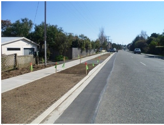
Aranui Road upgrade
