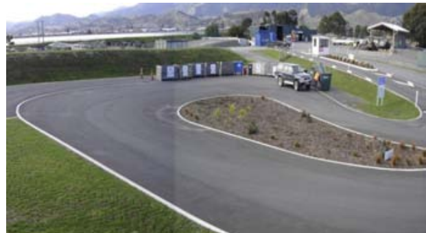
Richmond Resource Recovery Centre upgrade
