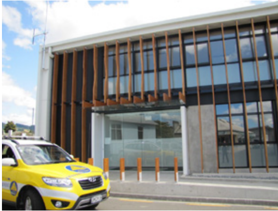
New Emergency Operations Building – Richmond
