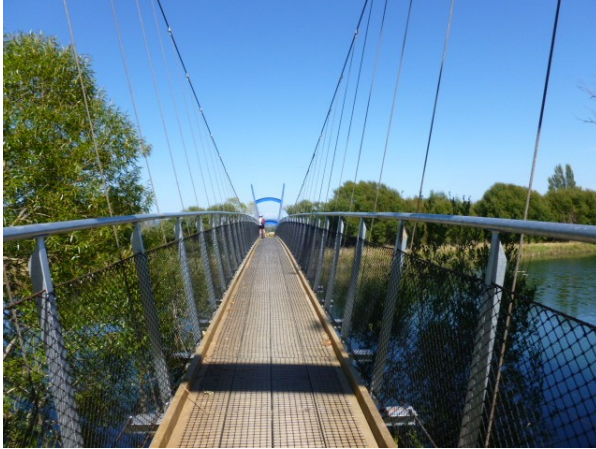
Cycle Bridge over the Waimea River
