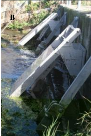
Figure 100: Retrofitted tidal flapgates showing the control arm connection with the tidal flapgate and headwall at low tide (A), the weight controlling the timing of opening at high tide (B), using weights to control the opening times (C) and a fish friendly tidal flapgate using a float (D); Photo courtesy of Kelly Hughes, Advanced Traffic Supplies.
