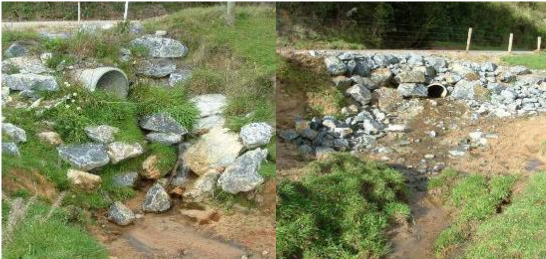
Figure 106: McShane Rd Culvert 23 before (left) and after (right)
