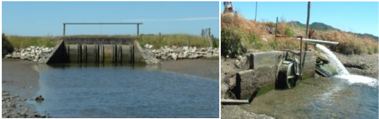
Figure 97: Left: Hamilton Drain near Riwaka (FP0412), right: North of Hamilton Drain near Riwaka (FP0850)
