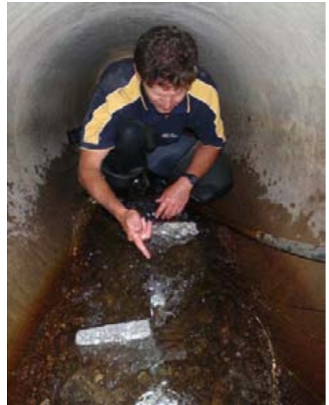
Figure 102: Stainless-steel baffles installed in culvert 25 in Wainui Bay
