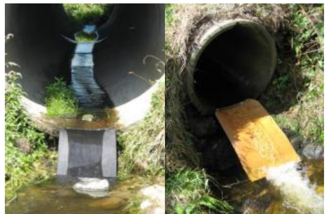
Figure 102: Stainless-steel baffles installed in culvert 25 in Wainui Bay
