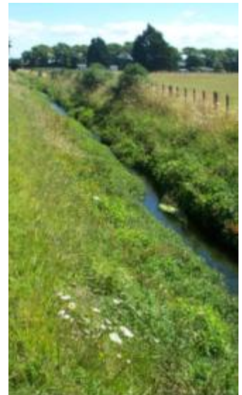
Figure 77: Borck Creek along Headingly Lane, Downstream
