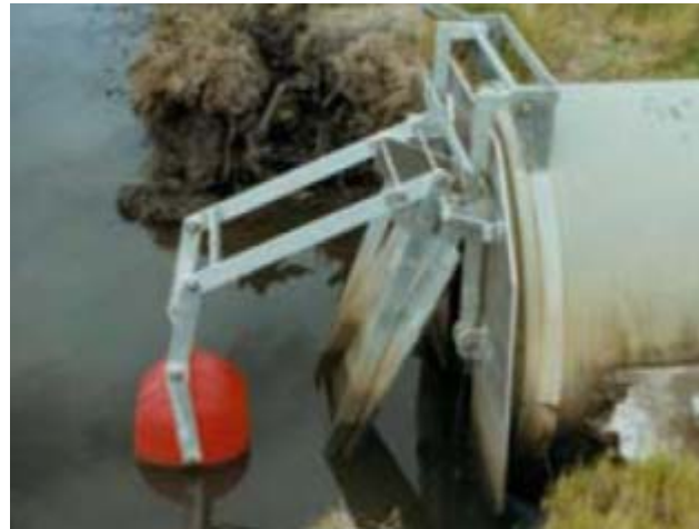
Figure 100: Retrofitted tidal flapgates showing the control arm connection with the tidal flapgate and headwall at low tide (A), the weight controlling the timing of opening at high tide (B), using weights to control the opening times (C) and a fish friendly tidal flapgate using a float (D); Photo courtesy of Kelly Hughes, Advanced Traffic Supplies.
