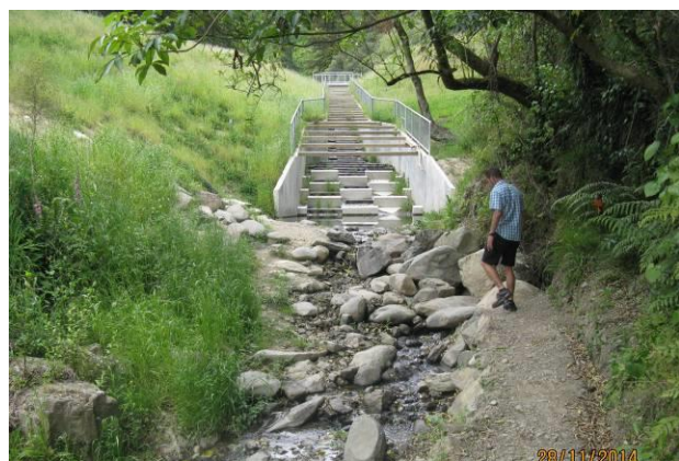
Reservoir Creek at the Reservoir Spillway (Nov 2014)
