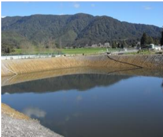
A dairy farm effluent pond; this pond has good storage and a weeping wall for solids removal
