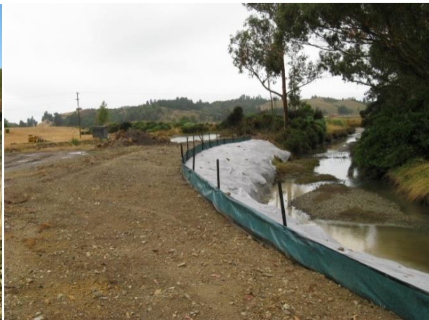
Silt fence for sediment control on flat terrain, Ford Creek, Tasman.
