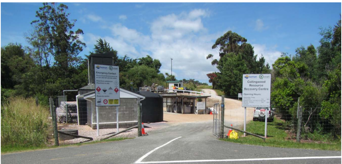
Figure B-8: Collingwood RRC – entrance from Collingwood-Bainham Road
