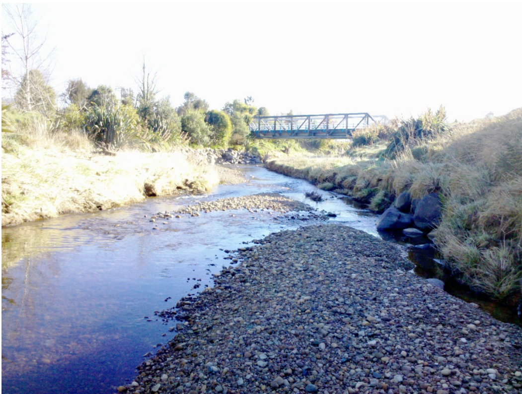
Figure B-6: Moutere River Looking Towards the Old House Road Bridge
