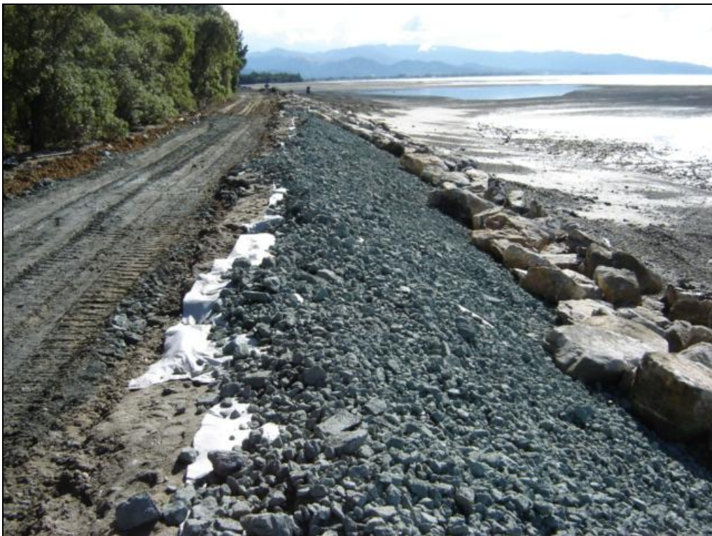
Kina Peninsula Road reinstatement progress
