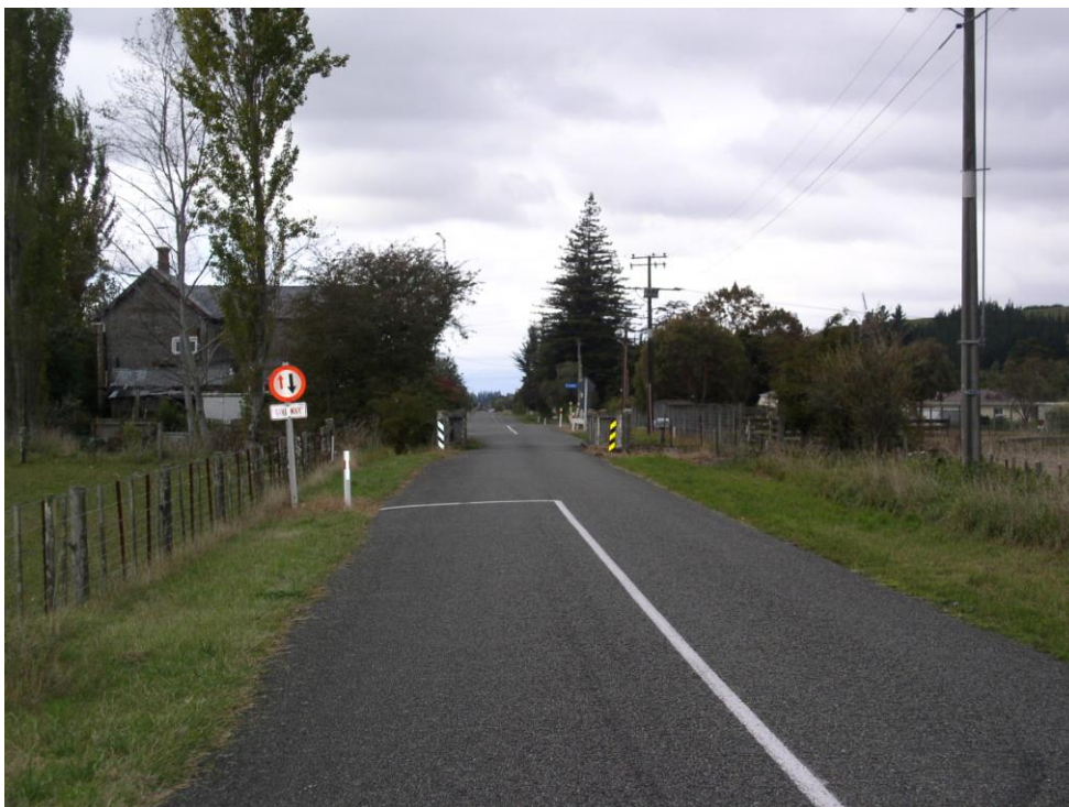
Telenius Bridge on Higgins Road – Looking North
