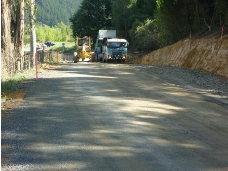
Eighty-Eight Valley Road
