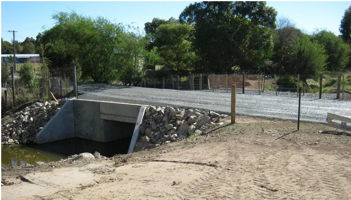
Recently installed culvert on Seaton Valley Stream
