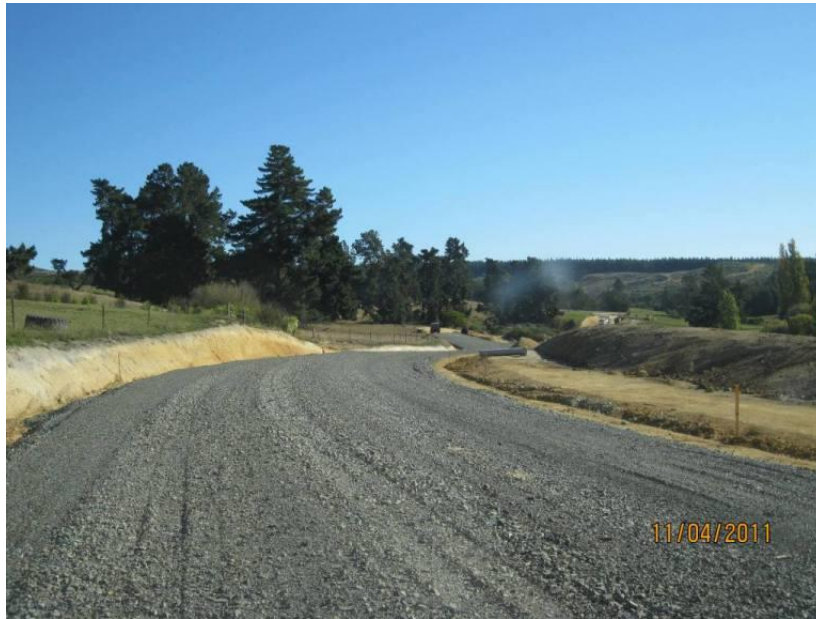
Section beyond Stn 700m with sub-base laid
