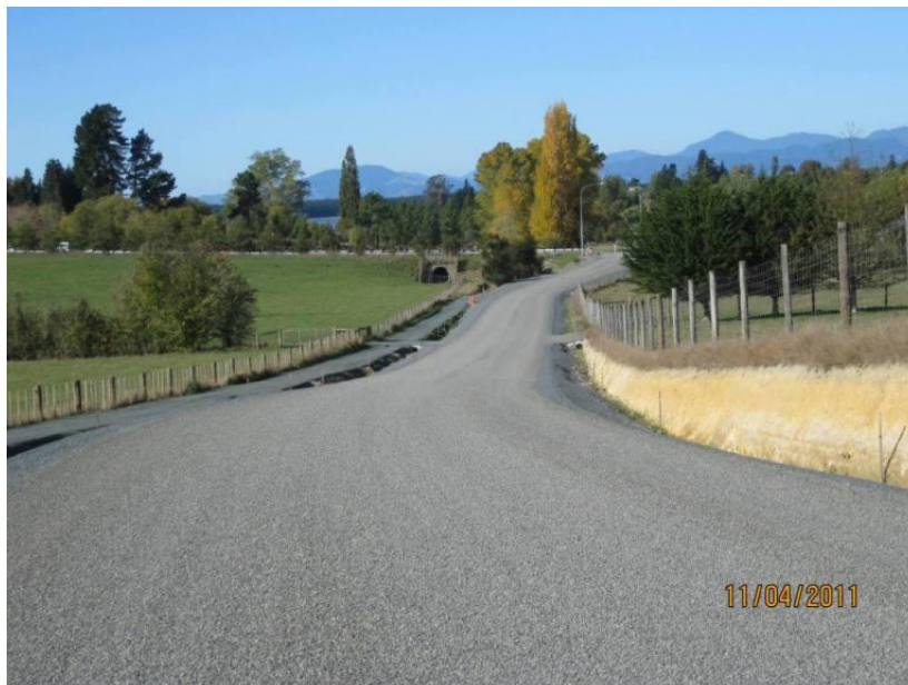
Stringer Road seal section from SH 60 to approximately stn 700m
