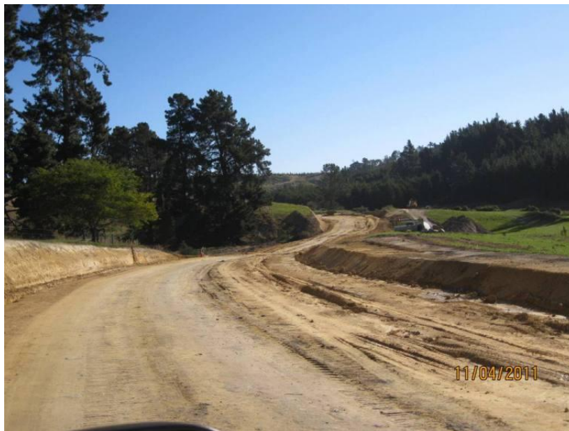
Earthworks formation to subgrade level on last section of Stringer Road
