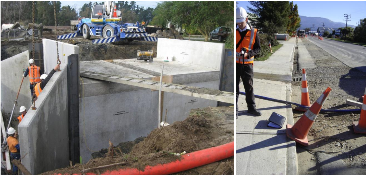
Installation of box culvert and new stormwater pipework
