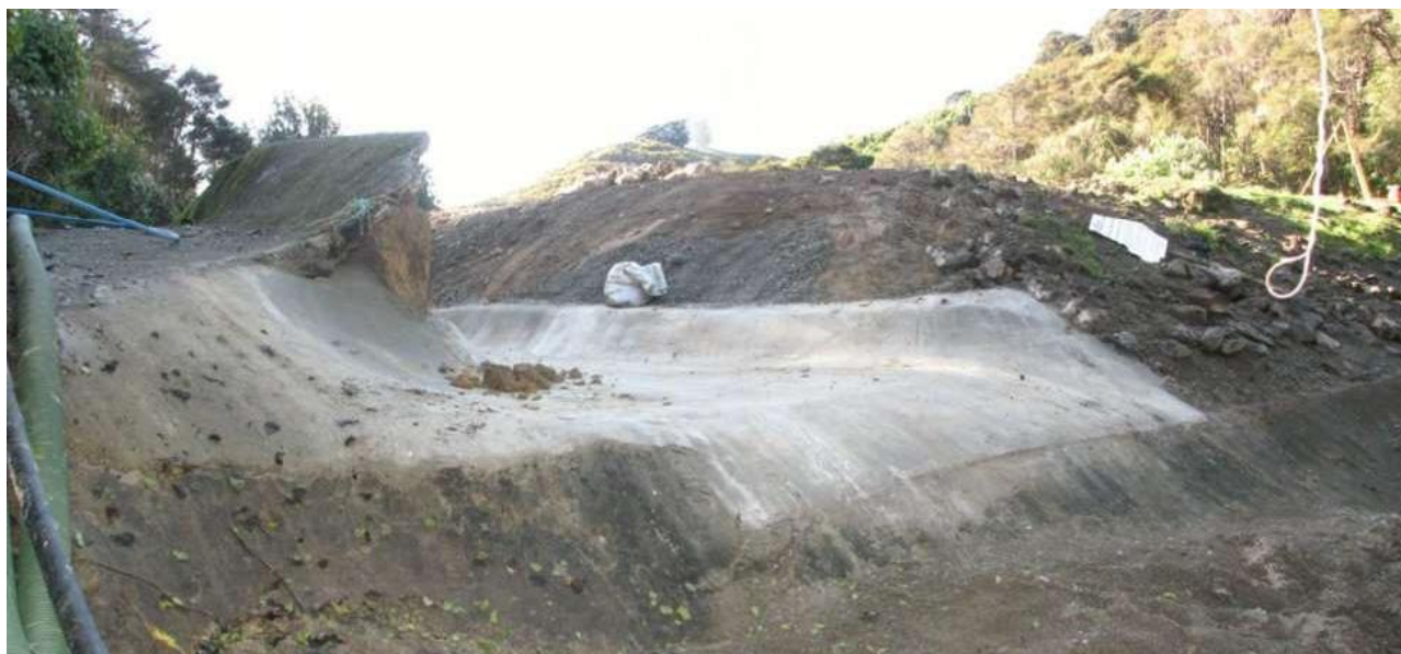
Construction of temporary spillway (Reservoir Creek Dam)
