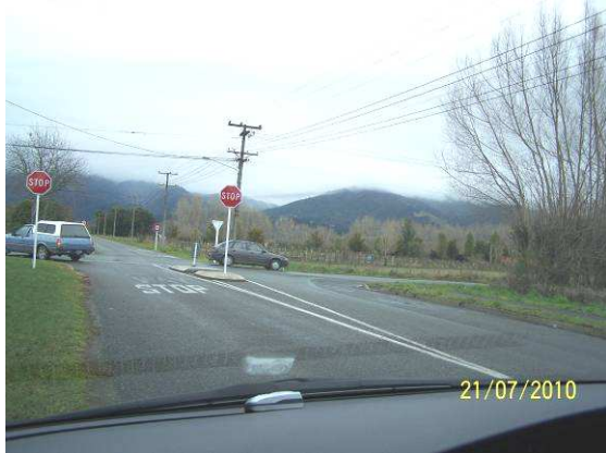
Photo 7: Low cost improvements, such as addition of splitter islands can improve intersection conspicuity.
