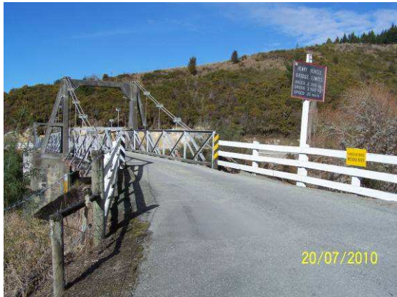
Photo 3: Posted structures may require more frequent inspection.
