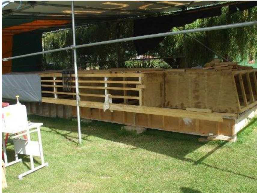
Ferry under construction – view shows it upside down
