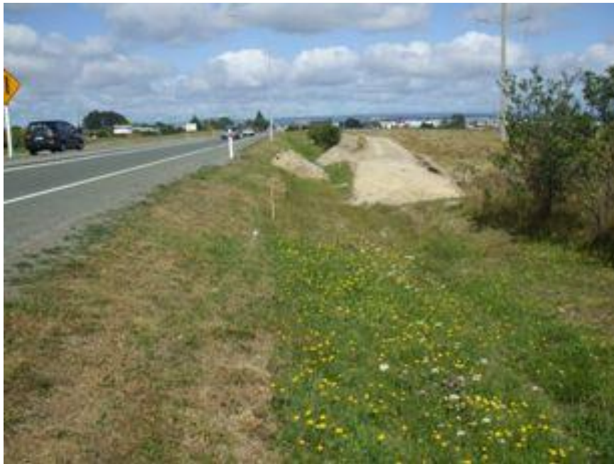
Richmond Deviation Cycleway – Construction commenced 10 January 2011
