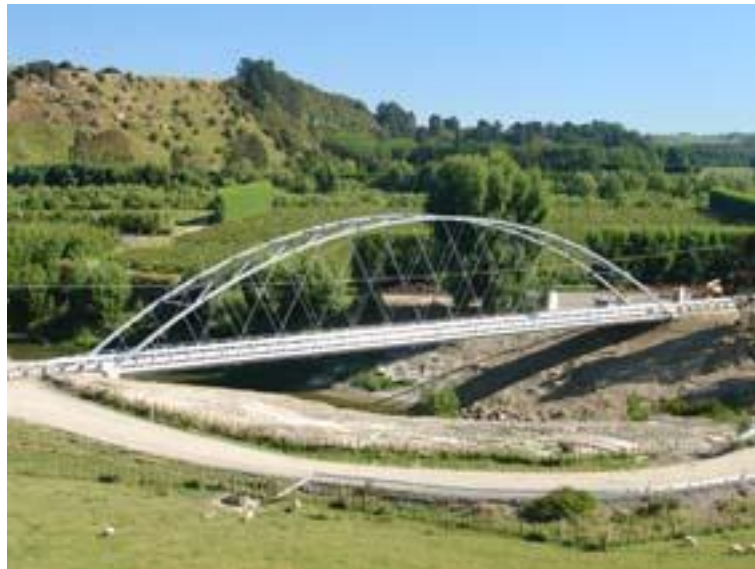
Photo of Network Arch Bridge (span 85m) in Wanganui District
