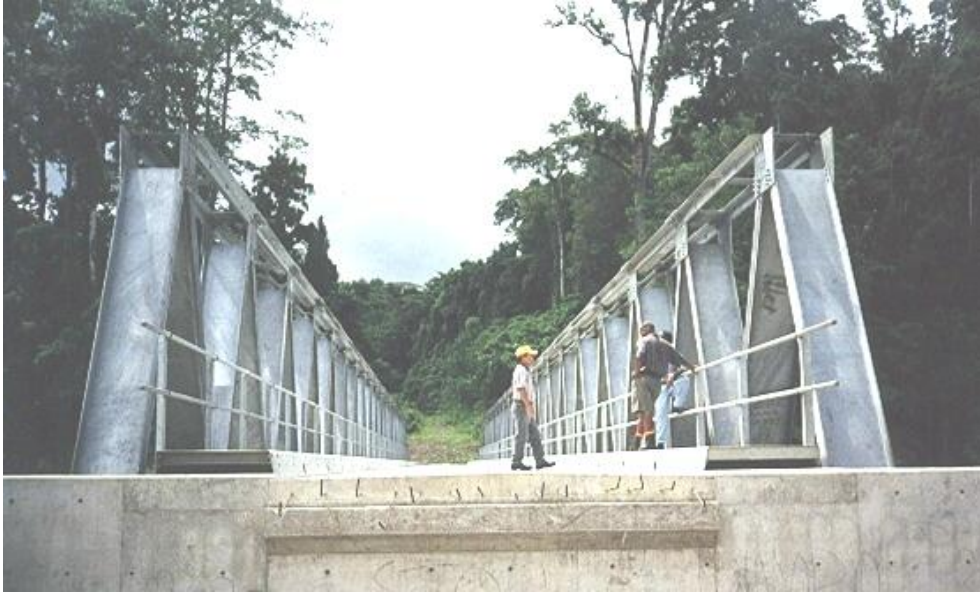
Photo of a Similar Thru Truss (this example had a span of 74m) This photo shows footpaths and handrails which have not been included in the Eastbridge estimate.
