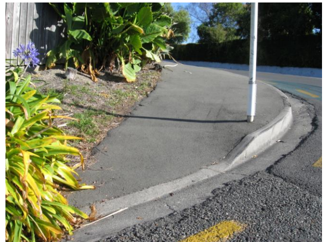
Pram Ramp on uphill southern side
