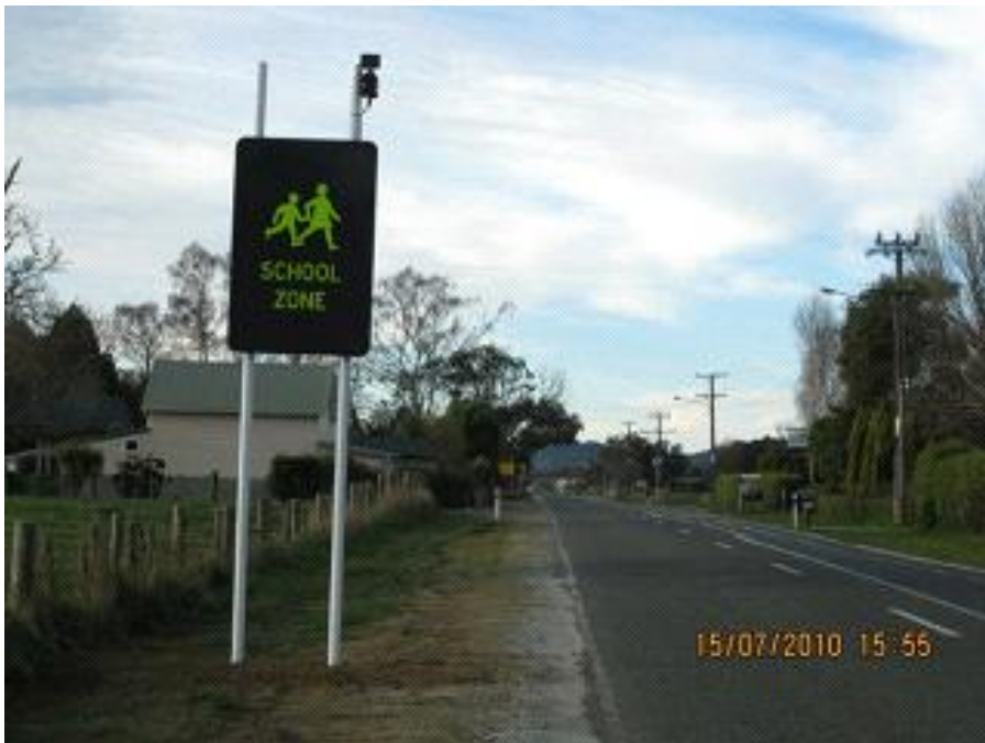
Active School Warning Sign outside Motupipi School
