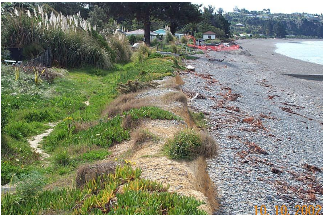
Photograph 1 - Coastal margin prior to construction of the revetment
