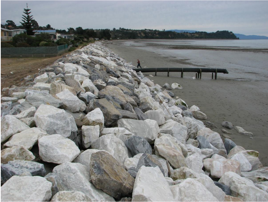
Photograph 3 - Existing rock revetment
