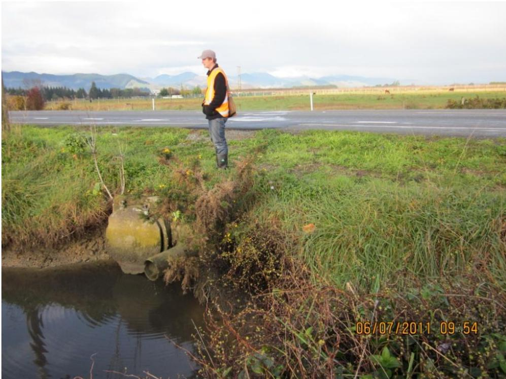
Photo 2: Location of where a platform or culvert extension and reclamation may be required to achieve adequate width.
