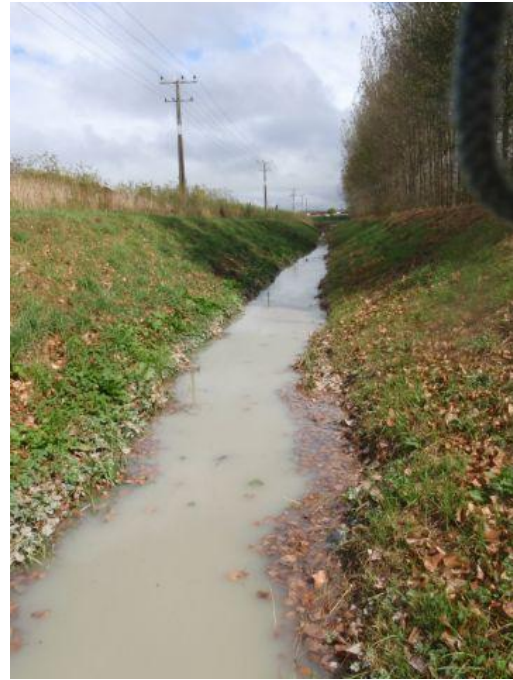
Borck Ck at Railway Reserve (upstream footbridge)
