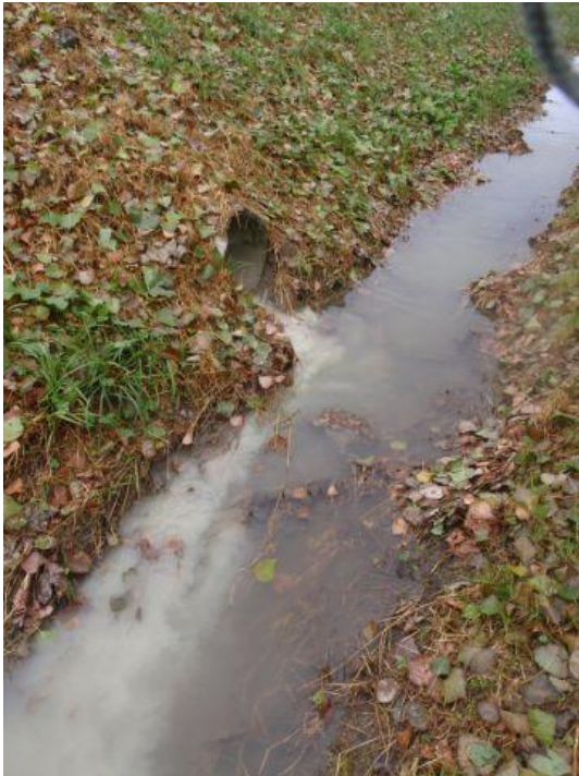
Figure 5a Discharge to Borck Creek downstream Gladstone Road on the Railway Reserve
