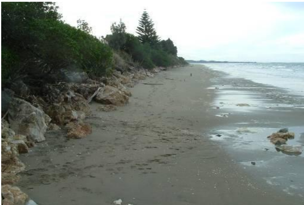
Photograph 1: Rock revetment at site
