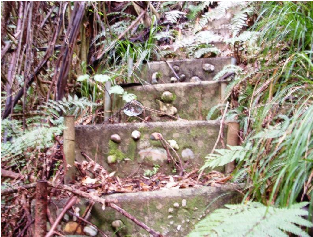
Photograph 3 – Part of the existing informal walkway
