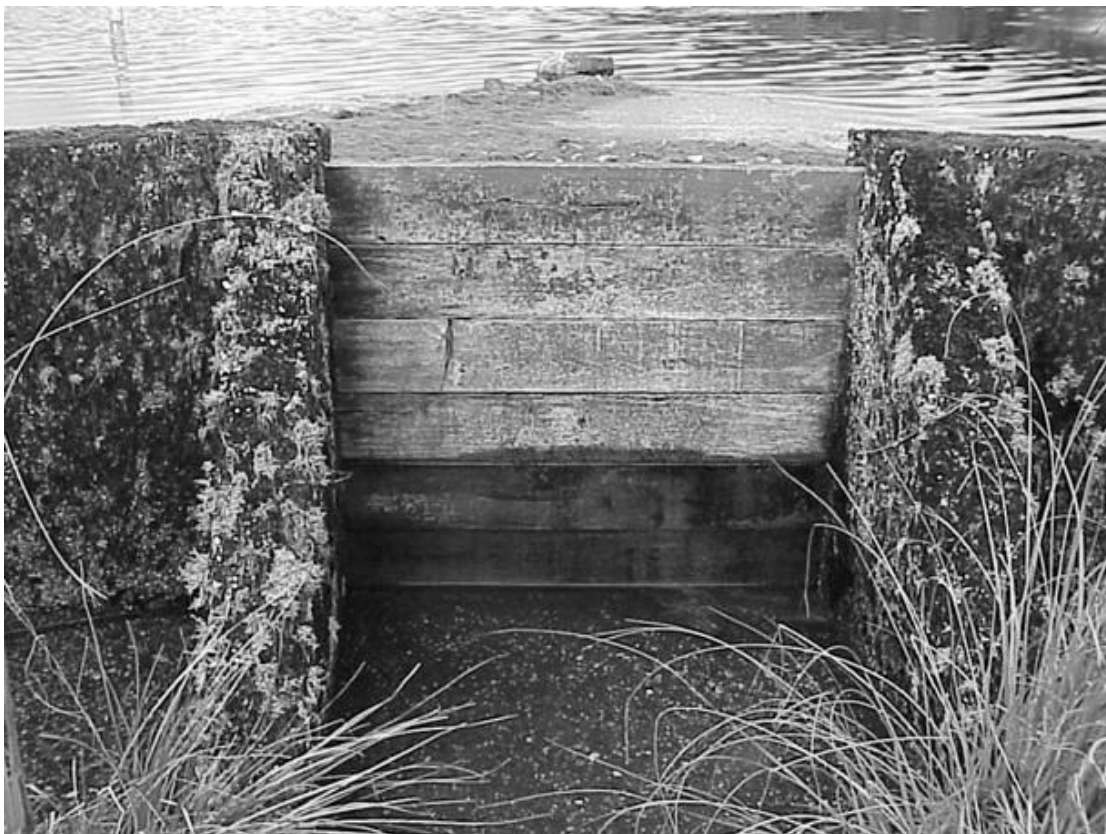
Example of a small weir.
