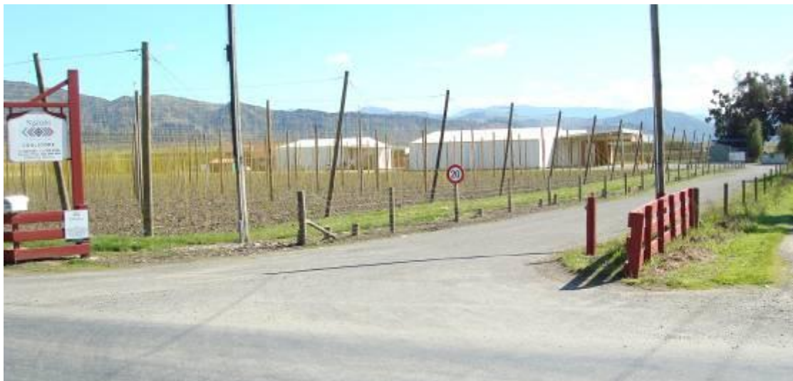
Photograph 2: Ngatahi Coolstores 278 Whakarewa Street Motueka
