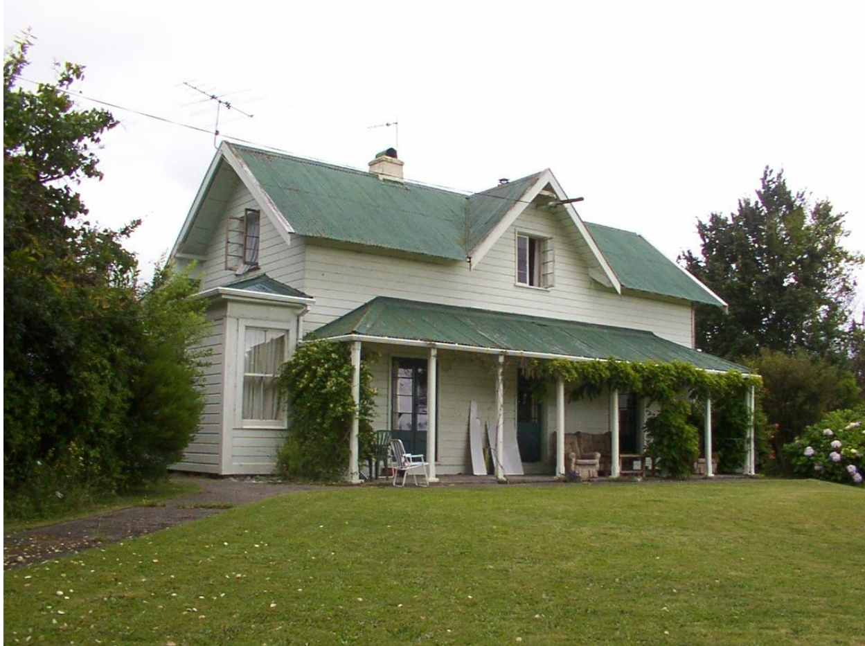
Photograph 4: Mr Whittakers residence. Heritage Building No 1668
