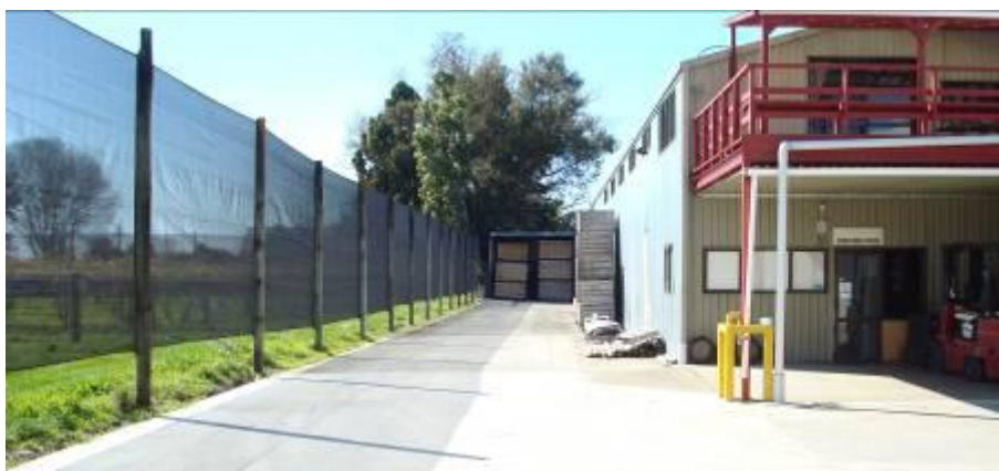
Photograph 3: View of vehicle exit access on north side of packhouse looking east towards Mr Whittaker's property Shadehouse (BC940306)
