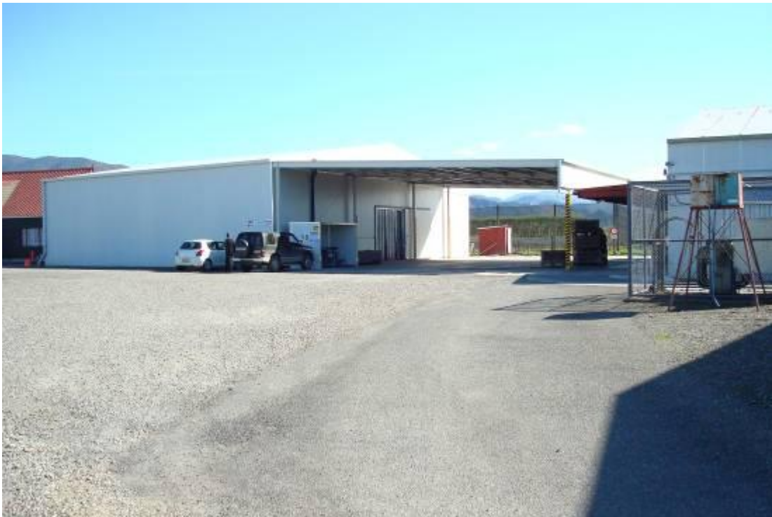
Photograph 11: Coolstore and canopy BC071627 (component E) with the main staff and visitor parking area on the left
