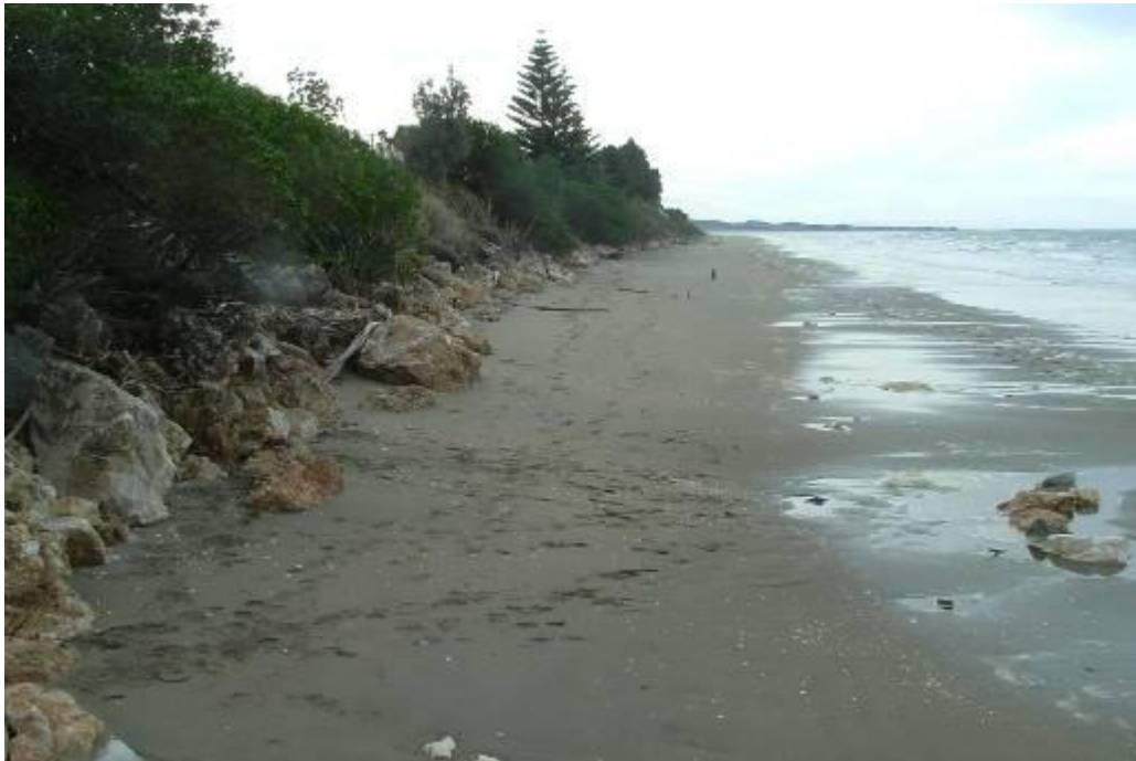
Photograph 1: Rock protection at site
