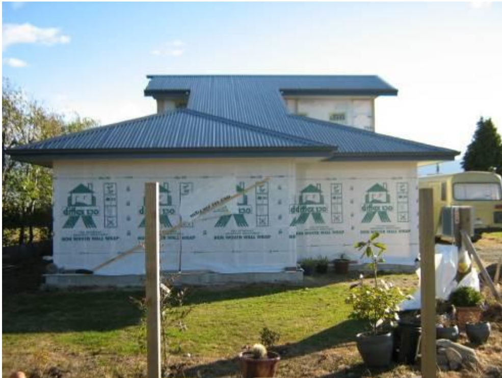
Figure 2: Photograph of the subject site looking west
