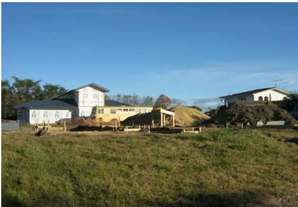
Figure 1: Photograph of subject site from Wharf Road
