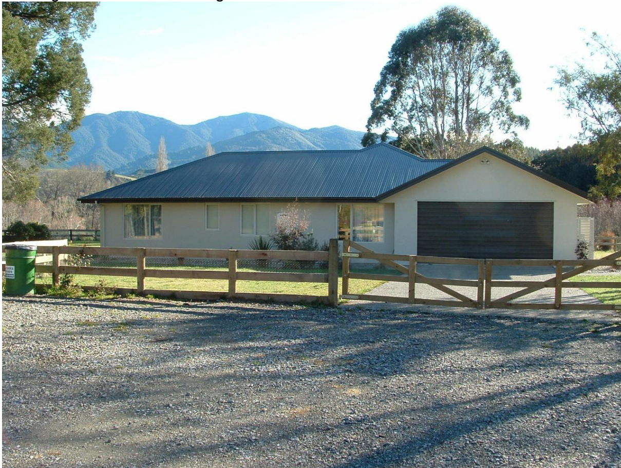
Existing house for farm manager
