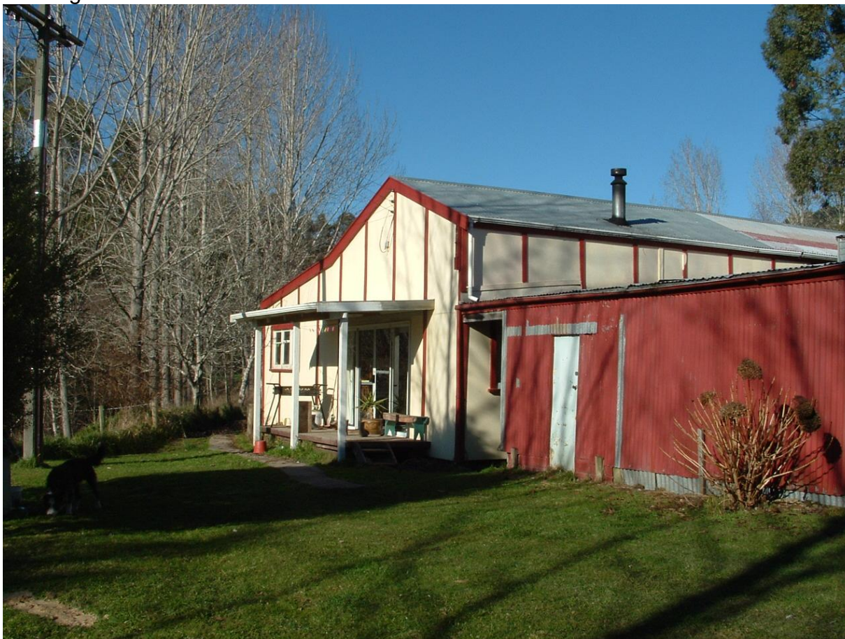
Existing workers' accommodation to be removed
