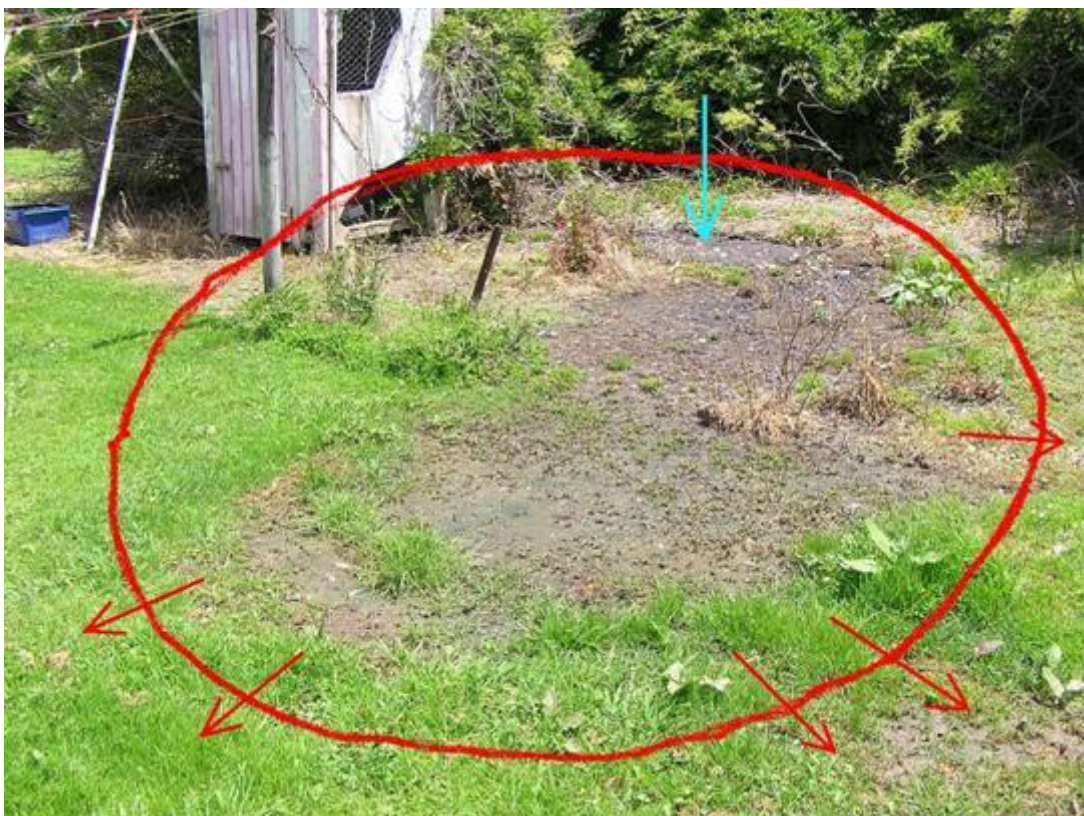
Rented accommodation: This septic tank has failed; note the surface expression of sewage at the point of the blue arrow flowing across the rear of the section in the direction of the red arrows. This system had been failing for some time, neighbours complained of the smell
