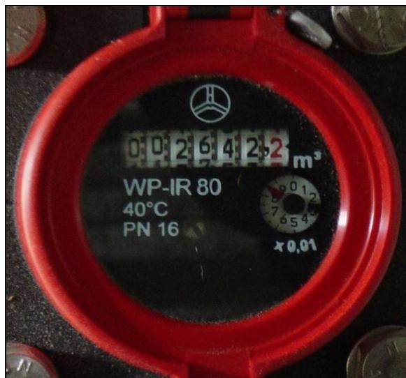
**Figure 2:** A New Style Meinecke Meter. Reading is 002642
