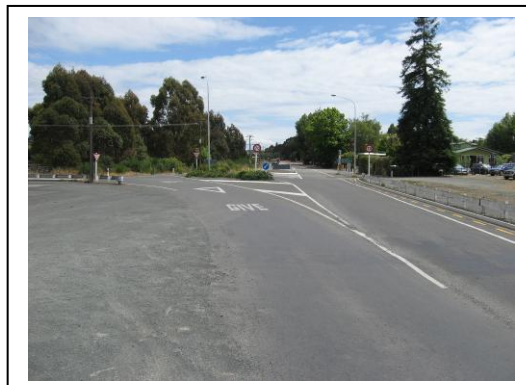
Photo 5: Aranui Road looking north towards SH60
