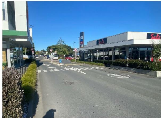
Figure 4-9: Incorrectly marked Pedestrian crossing
