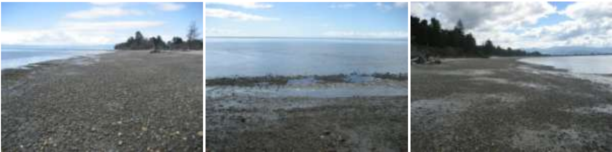
Erosion at the southern end of Jackett Island
