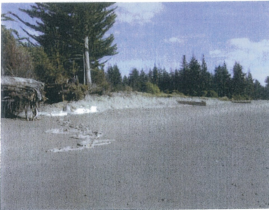
Photograph 3 - existing shoreline showing two timber groynes (8 April 2011)
