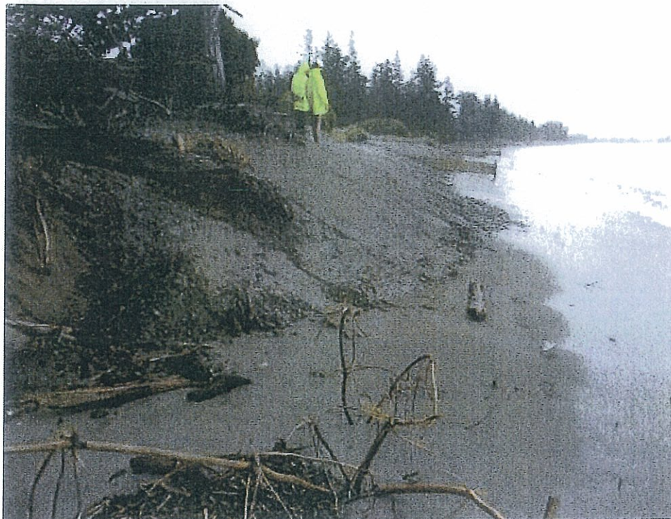
Photograph 1 Completed emergency works as at 6 July 2011
