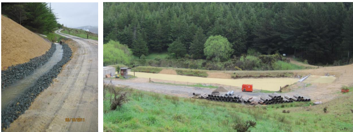
Eves Valley Landfill stormwater improvements
