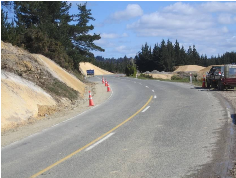
Moutere Hill Shoulder Widening
