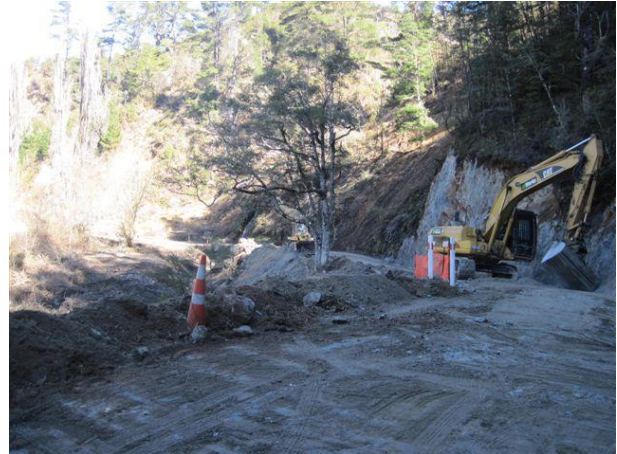
Widening at Baton Valley Road
