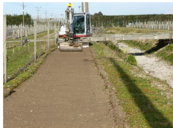
Railway Reserve through Waimea Estate
