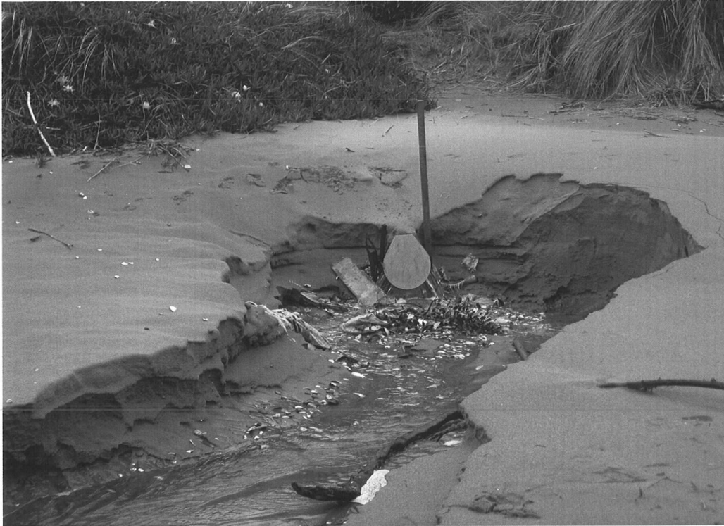
DRAIN ALONGSIDE RESERVE TRACK SEPT 29 CLEAR FLOW TO SEA
