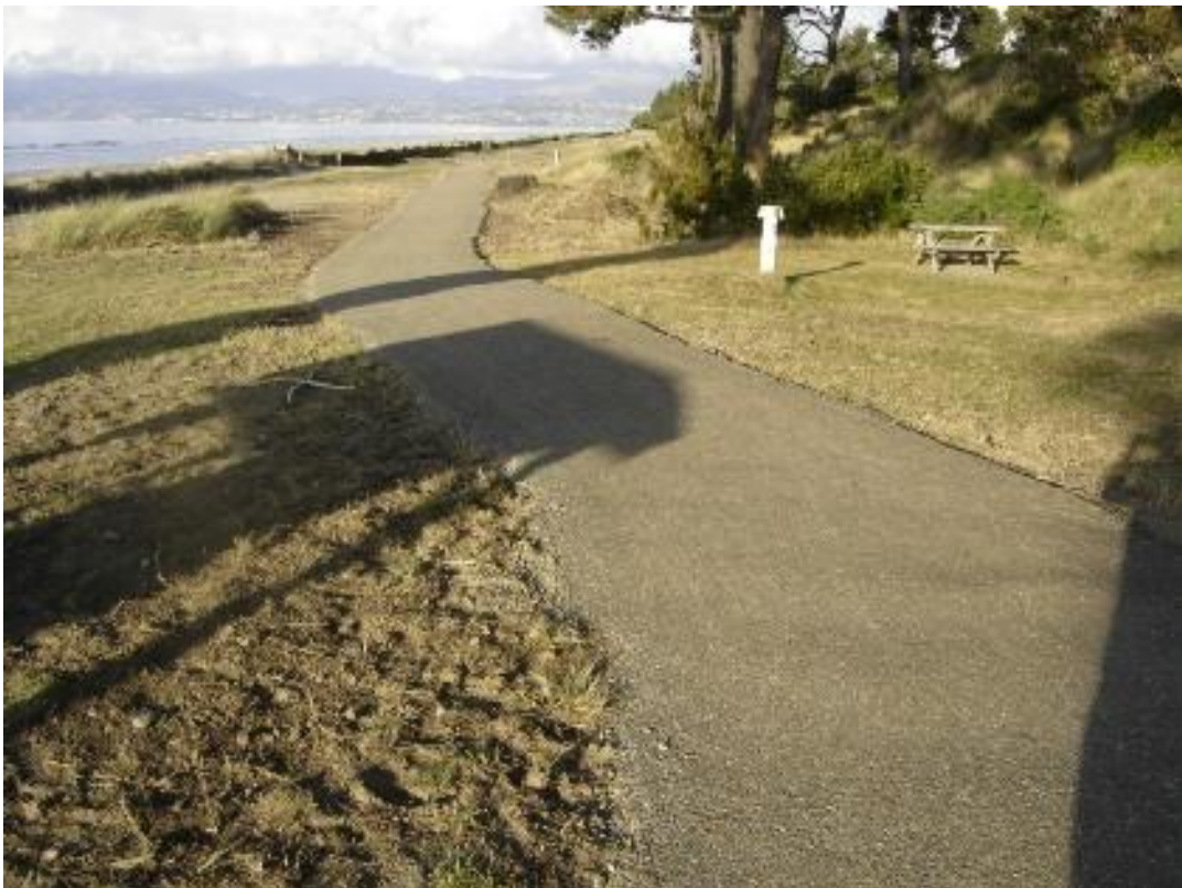
Rabbit Island Frontage – Completed trail
