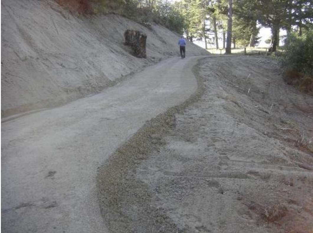
New trail at Rabbit Island – partial construction
