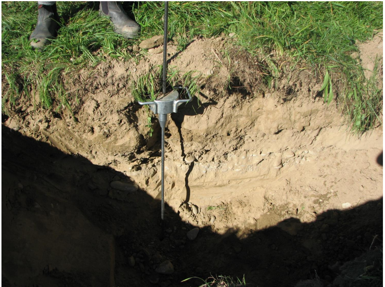
Figure A3: Test pit in crest of existing stopbank (TP07A)
