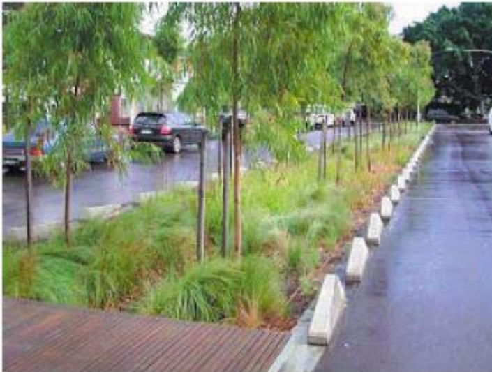
Figure C3a Rain garden in a residential street
