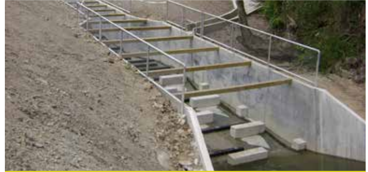
New spillway with 'fish ladder'
