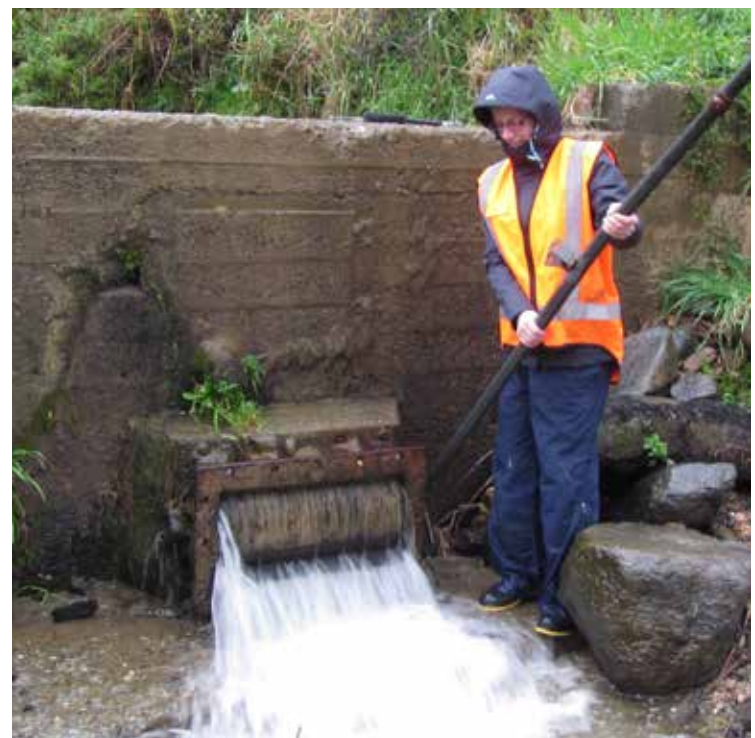
Dr Gill Bullock opening a scour valve at the Pohara water supply intake
