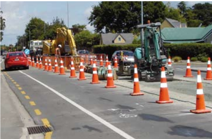
Work underway on Salisbury Road.
